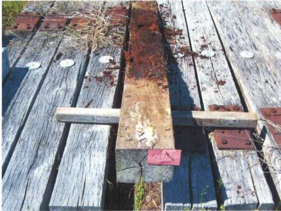
Figure 43 - Tie #203 (Cedar-cide/red oak) with decay.
