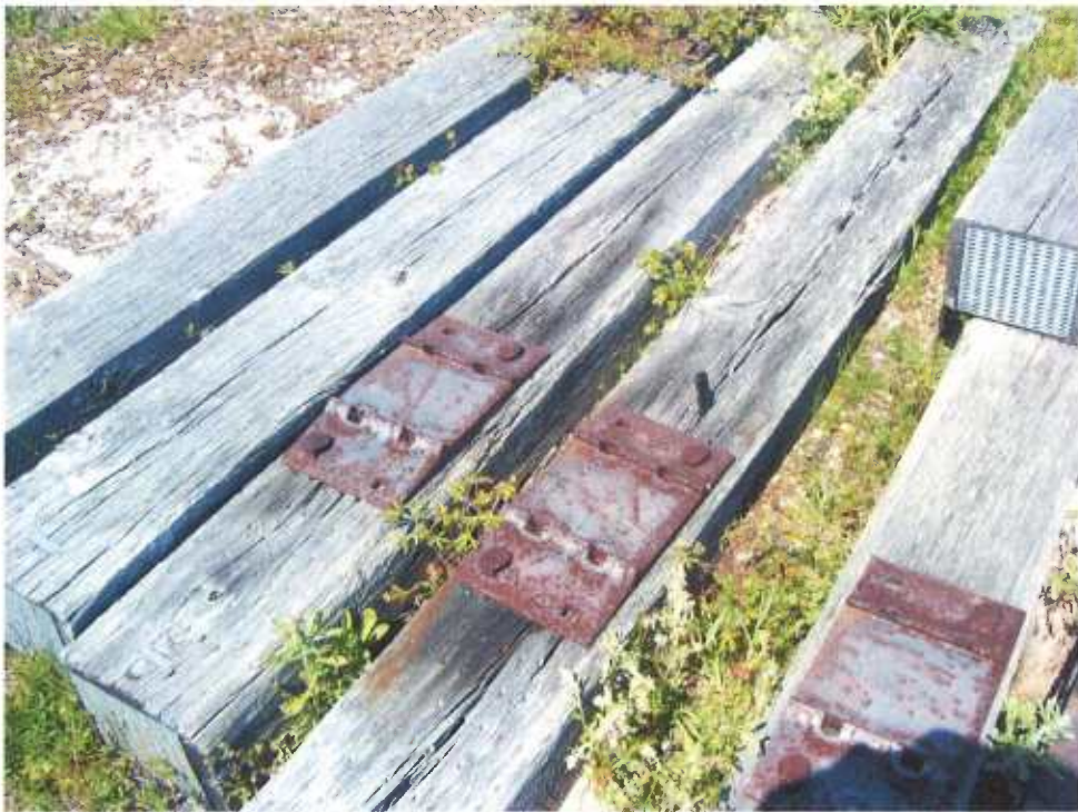
Figure 6 - Tie #334 with checking, decay and "iron sickness".
