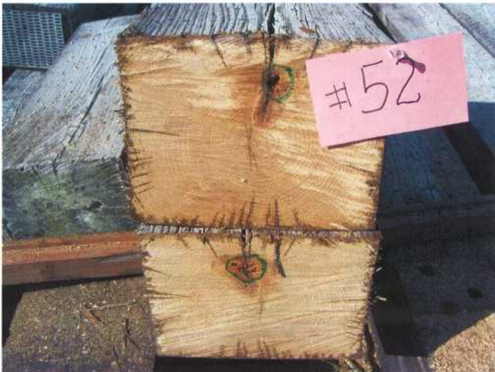
Figure 12 - Tie #52 (Boatright/white oak/creosote to refusal) decay around check.
