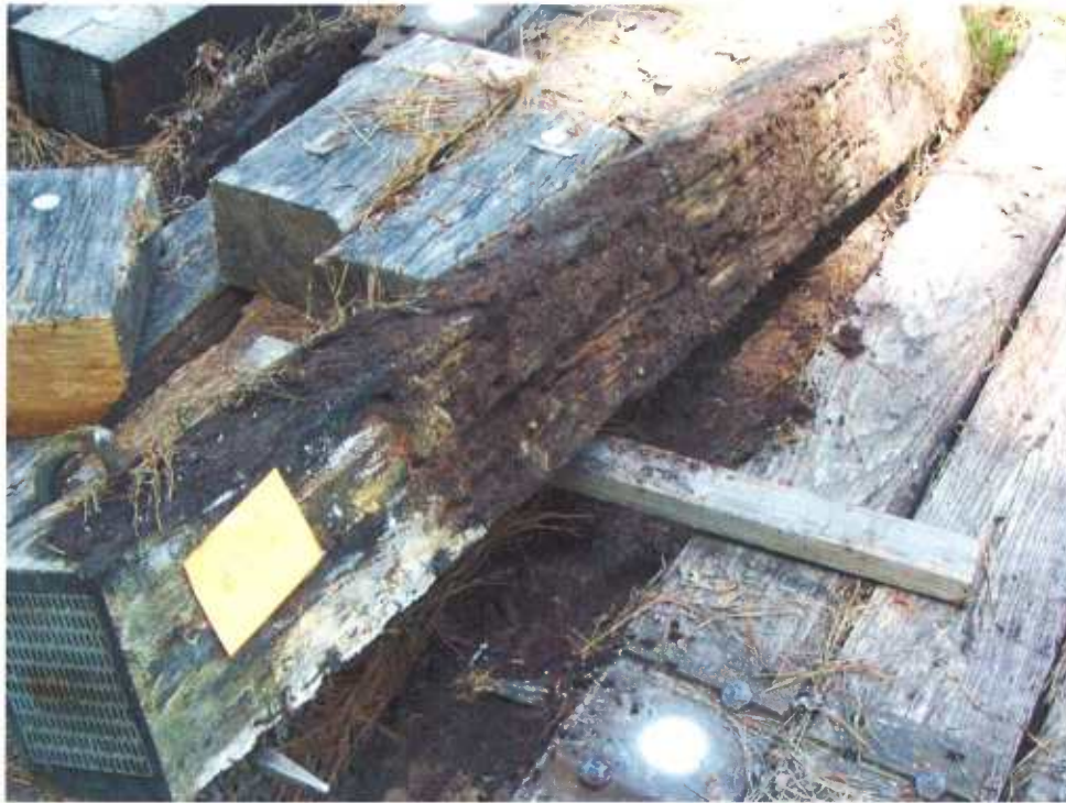
Figure 35 - Tie #172 (red oak/control) with heavy decay on bottom.
