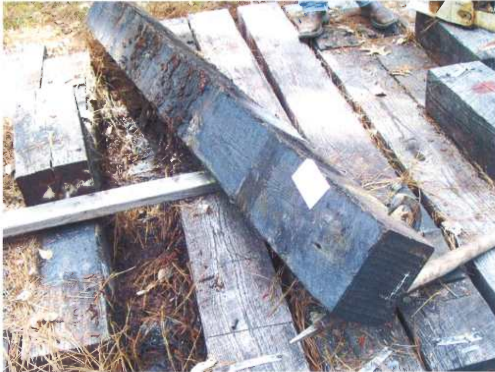
Figure 7 - Tie #39 (Boatright/red oak/borate/creosote 7pcf).
