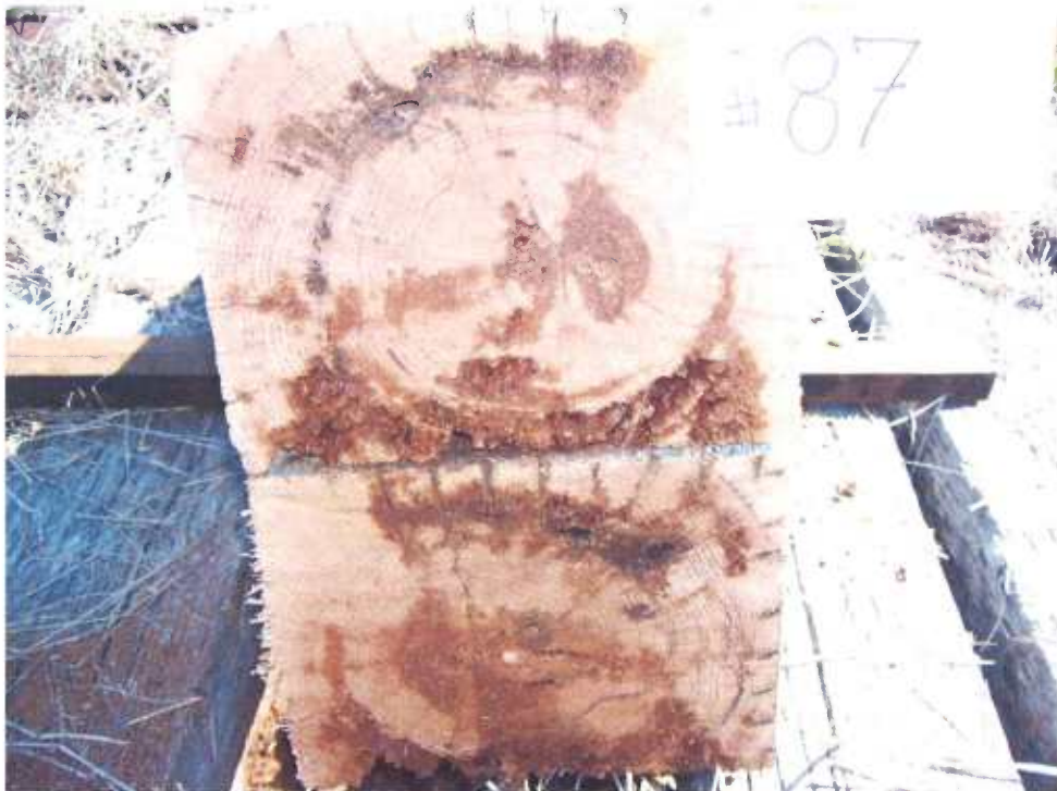
Figure 18 - Tie #87 (Lonza/red oak) decay evident in cross-section.
