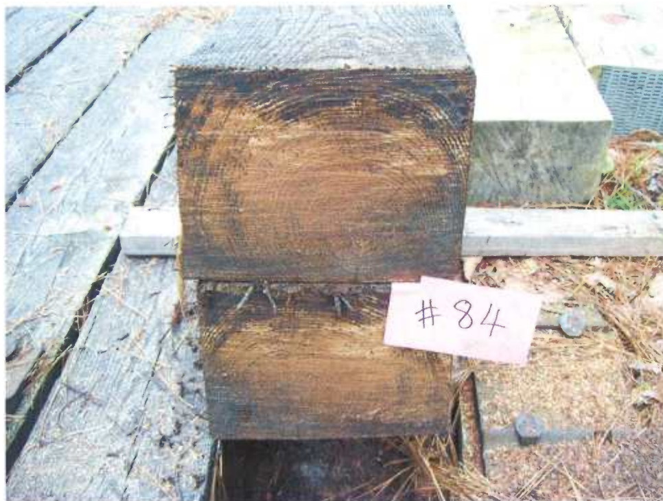
Figure 16 - Tie #84 (Boatright/red oak/borate/creosote 5pcf).
