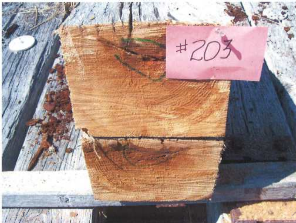
Figure 44 - Tie #203 (Cedar-cide/red oak) with decay in cross-section.
