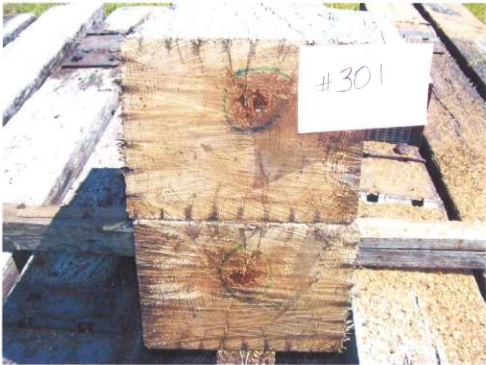
Figure 60 - Tie #301 (Koppers/red oak/creosote petroleum) with decay in cross-section.
