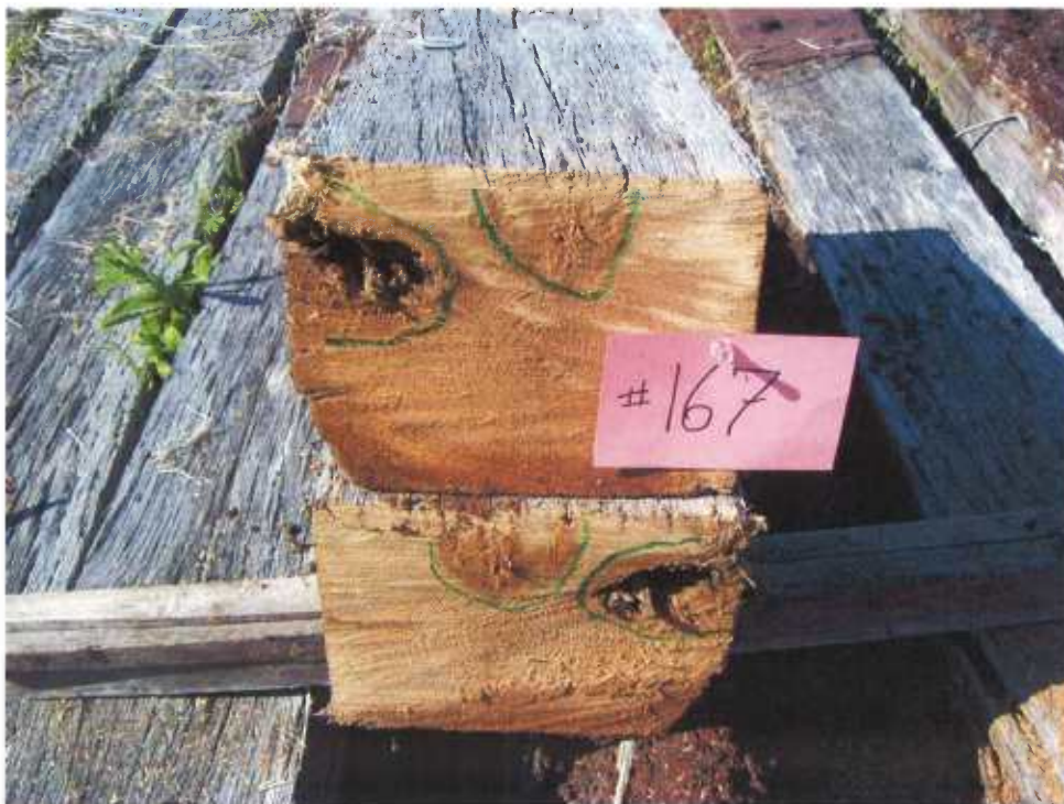
Figure 34 - Tie #167 (white oak control) with decay evident on all surfaces.
