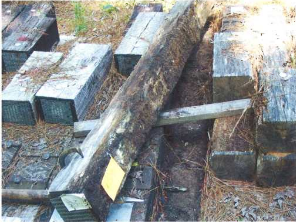
Figure 33 – Tie #169 (white oak/control) with light decay and fruiting bodies.
